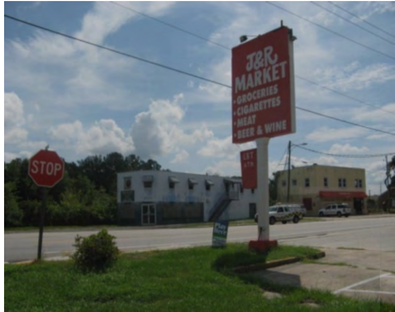
Example of commercial buildings in the VRSA. On Baxter Street looking southeast at Spruill Avenue.
