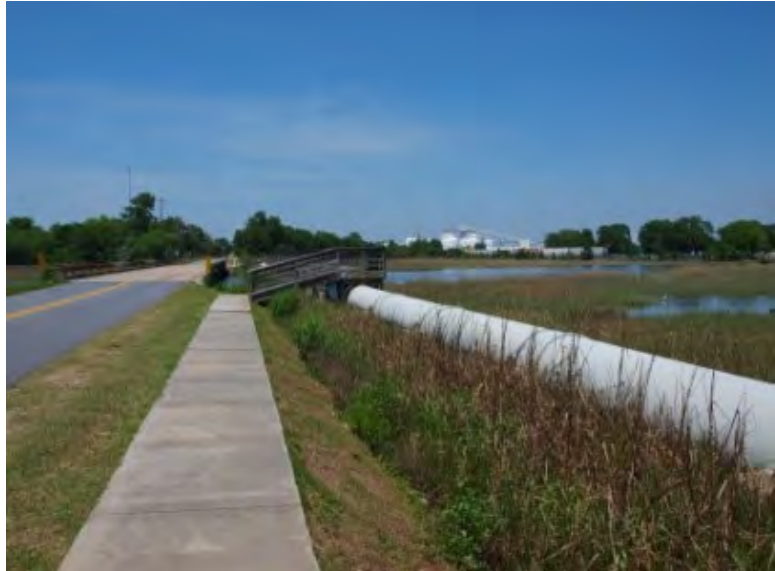
Looking north on O’Hear Avenue over Noisette Creek at built structures.
