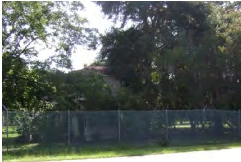
Sample view of vacant housing on River Center project site.
