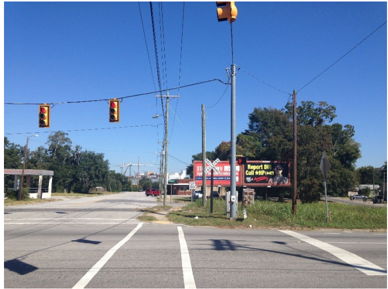
View east from Chicora-Cherokee neighborhood west of Spruill Avenue down Reynolds Ave
